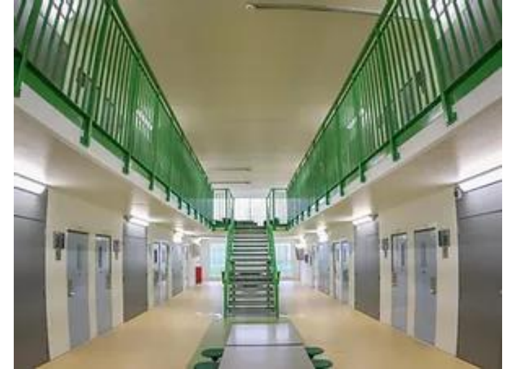
Typical internal prison welded / fabricated steelwork
